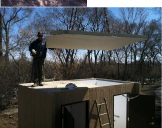
3. Ceiling Panels The ceiling panels will have four liftings hooks to lift and set in place. Make sure the vents are lined up with the angled corner. When the panels are in place use the white caulking to seal the inside seam between the ceiling panels and the wall panels.
