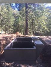
The body is set on the vault with the back and side walls flush with the vault. The septic tape will make a water tight seal.
